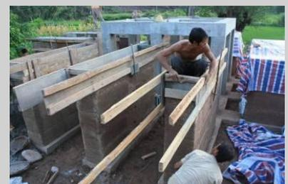
Testing of anti-seismic rammed earth construction
